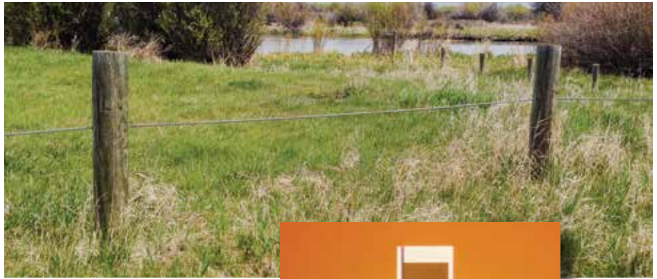
Above: A low post and single cable or chain fence creates little hazard to wildlife if it can be easily seen.
