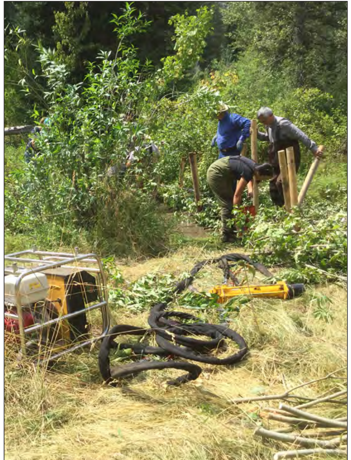
Hands-on Training. NRCS staff learning how to build beaver dam analogues at a workshop in Utah. Photo by Jeremy Maestas.
